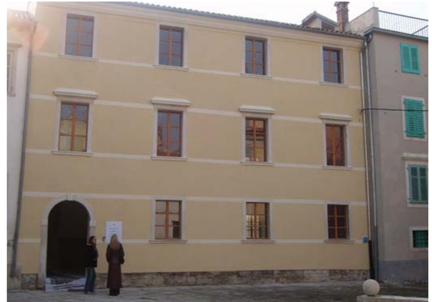
The "Fishermen's School," Piran, late eighteenth century. Originally built as a crafts school, the building has housed the Piran office of the Institute for Mediterranean Heritage since its renovation in 2005 Photograph: Institute for Mediterranean Heritage
